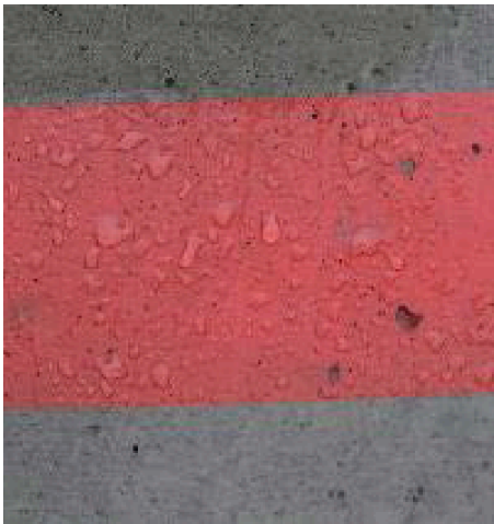
Figure 2. Colouration and protection of GRC
